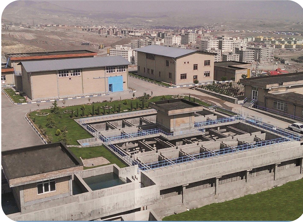
PARDIS City Water Treatment Plant
