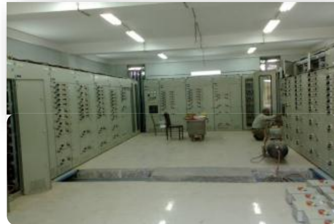
FARABI Sugar Refinery Factory Equipment installation & Startup
