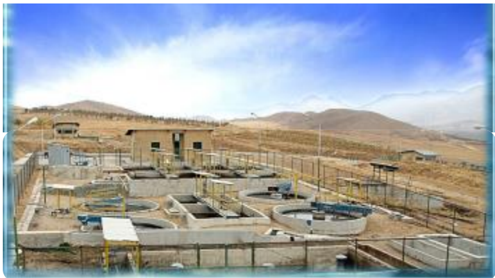
SHAHR-E-KORD Slaughterhouse Wastewater Treatment Plant
